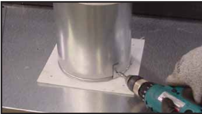
Figure 9.7 To attach the first section of vent pipe, make sure to use the fiberglass gasket in the manual bag to seal between the first vent component and the outer fireplace wrap. Use 2 self tapping screws to secure the gasket to the outer wrap.
