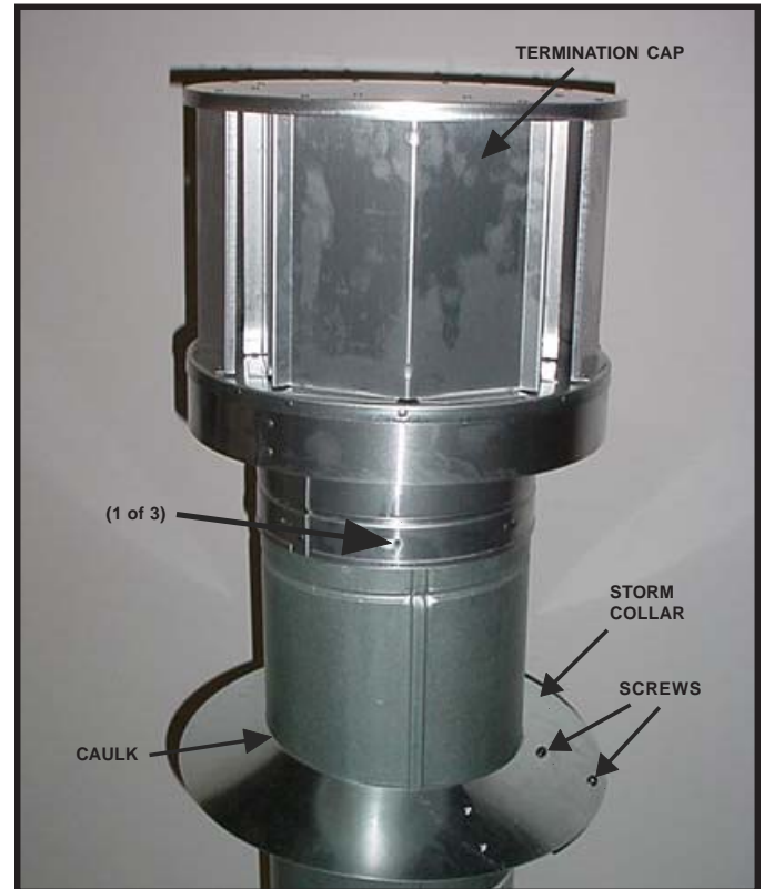
Figure 8.14 Termination Cap - DVP-TVHW
