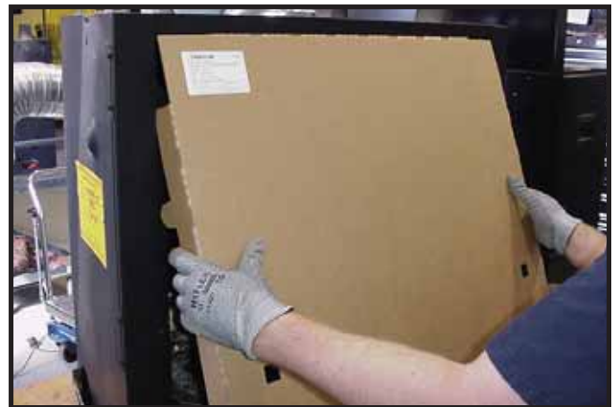
Figure 13.4 Installation of Splatter Guard
