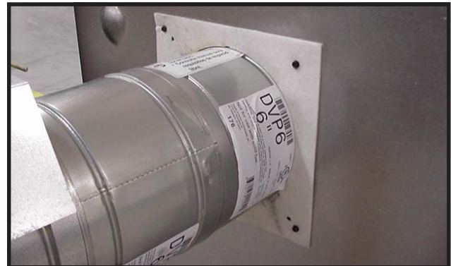
Figure 27. Attach the first flue section (it will snap into place). Slide the insulation gasket onto the flue section, up against the appliance and over the tabs. Use two self-tapping screws to secure gasket to outer wrap.
