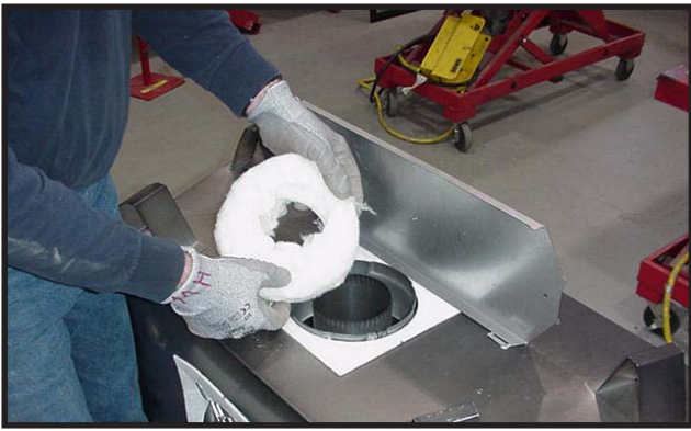
Figure 21. Remove the insulation from the outer flue pipe.
