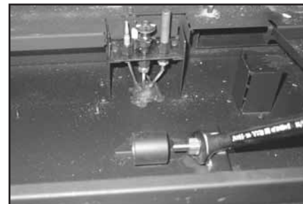
Figure 6.3 With a 5/8 in. wrench remove orifice retaining nut. Replace with appropriate orifice.
