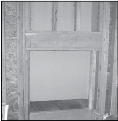
Figure 13.1 Sheetrocked Chase
