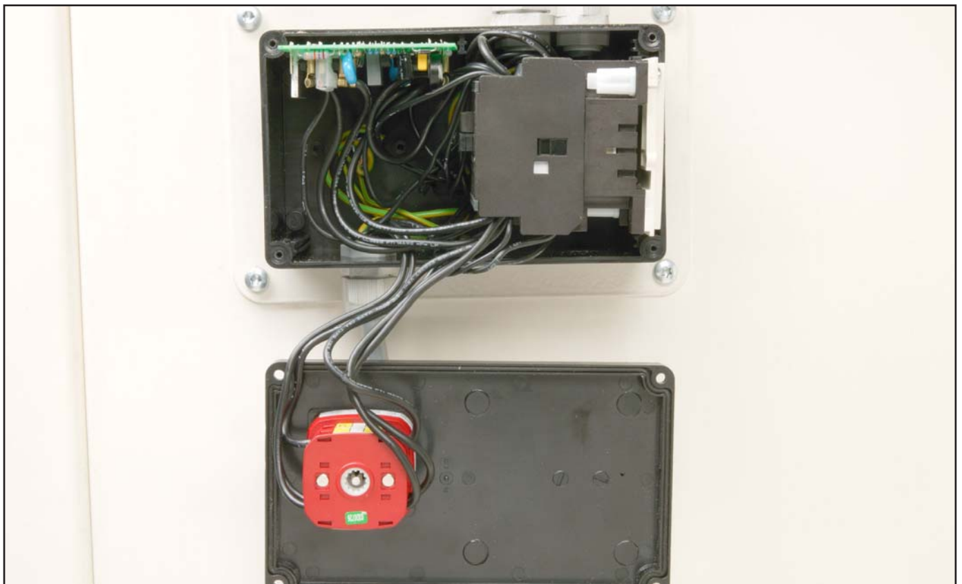
Figure 101. Main switch box wiring.
