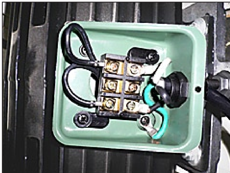
Figure 39. Motor Junction Box.
