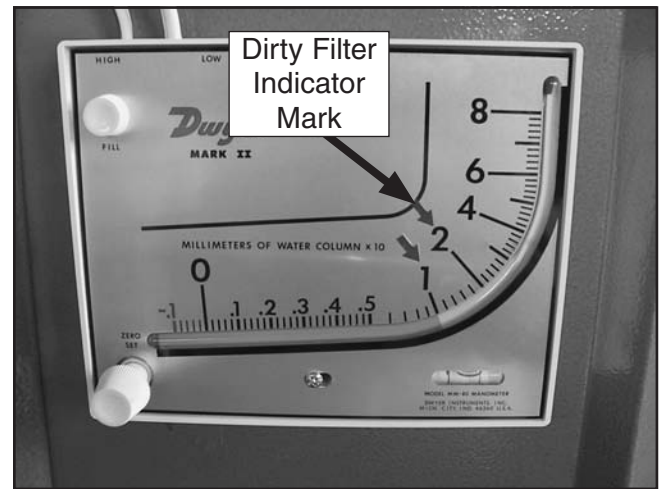
Figure 20. Dirty filter mark example.
