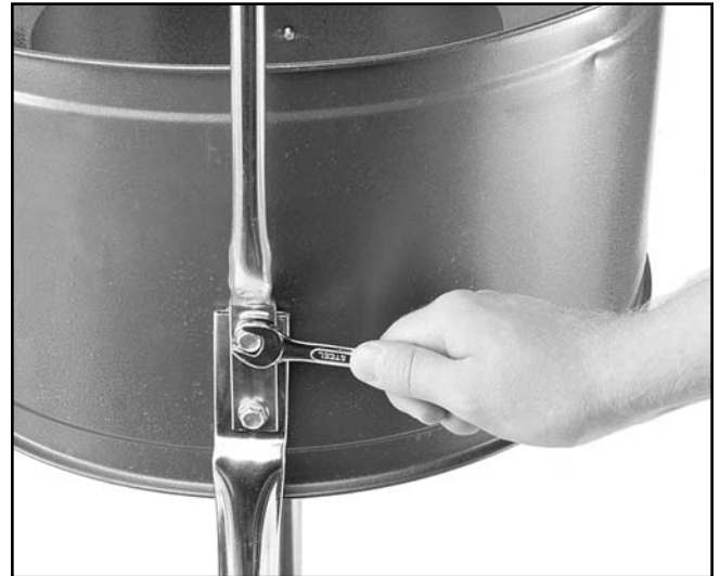
Figure 6. Mounting collector to brackets.
