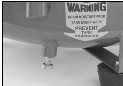
Figure 5. Drain valve location.
