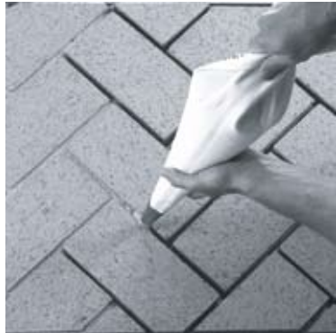
Figure 20 - Grouting Brick INSTALLING SCREEN
