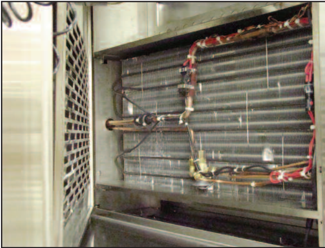
Evaporator Coil
