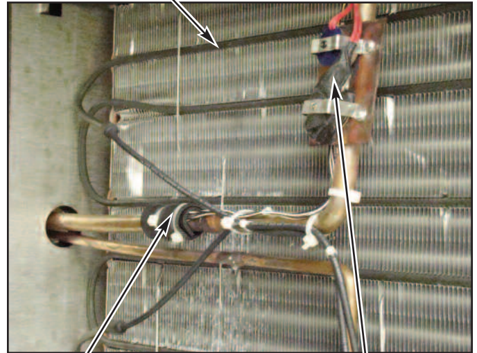
Coil Sensor - SN-33541
